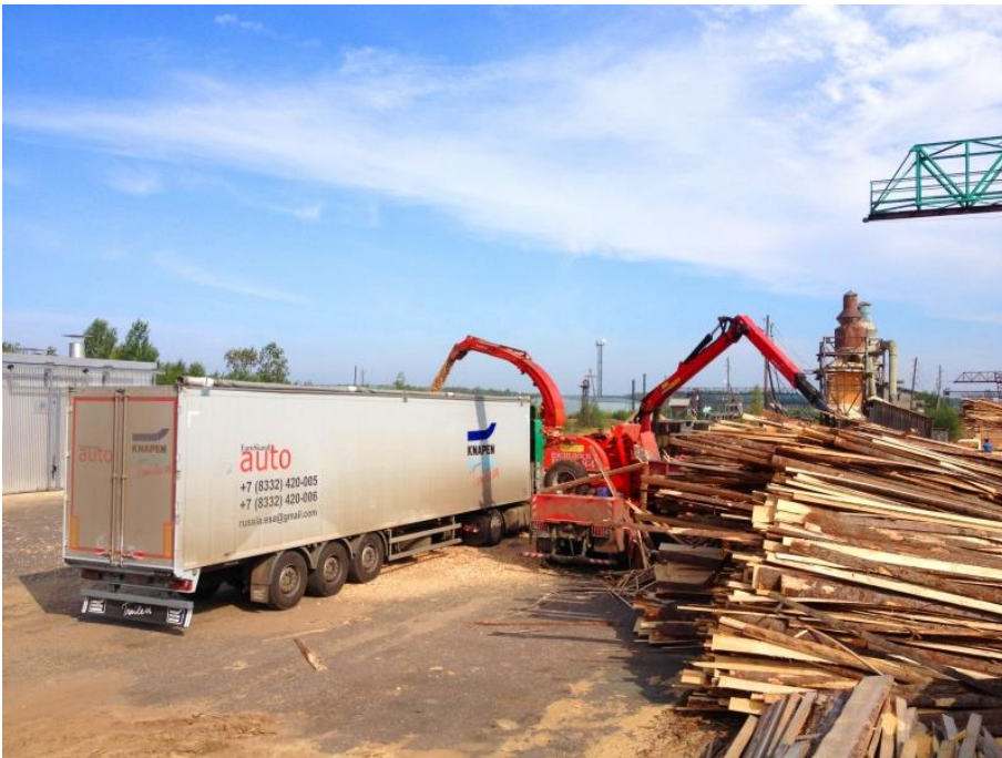
Picture: Loading a moving floor on site. Be aware of the danger zone
