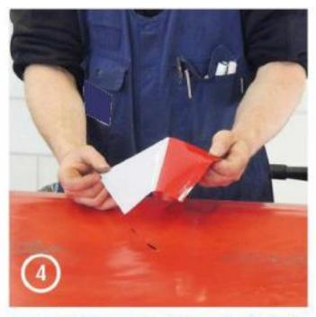
Remove the transparent film on the back of the tape
