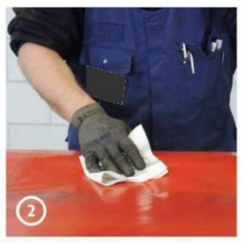
Make sure that all dirt, grease, oil, etc. is removed from the surface to be repaired Ensure that the surface is completely dry before applying the tape
