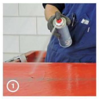
Carefully clean the area to be taped with a grease-free and silicon-free cleaning agent
