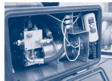
Figure 2.3.2.e. – Electrohydraulic unit with operating button
