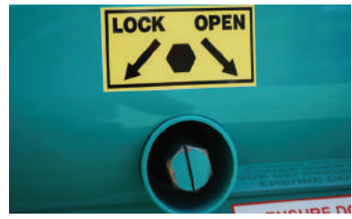
Mechanism to open or close partition doors
