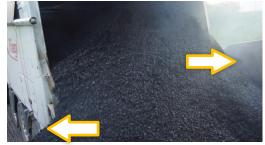
Fig. 62: Excessively fast push-off process
